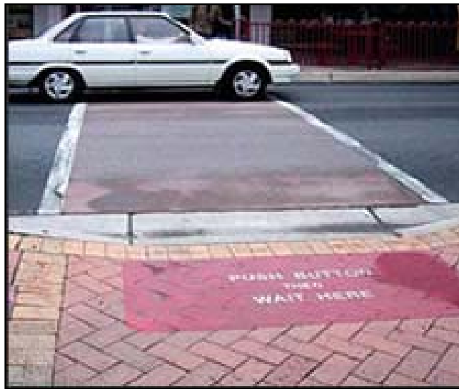
Figure 8: Australian piezoelectric sensor in a sidewalk under red painted area.
