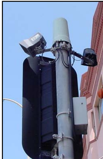
Figure 6: Infrared detectors in Sydney, Australia.
