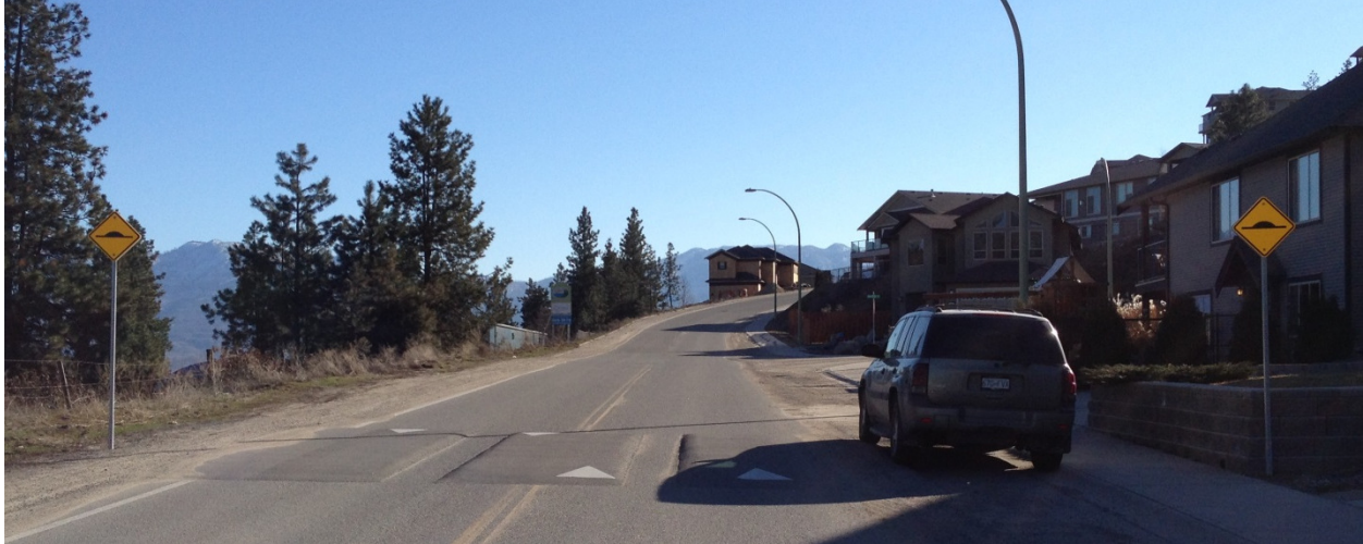
Figure 4 – Speed Cushion on Auburn Road
