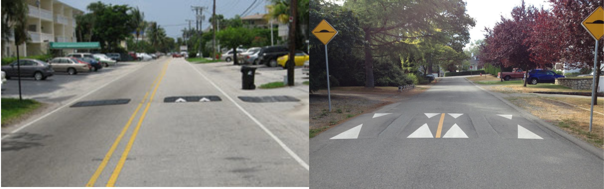
Figure 1 – Speed Cushion Layouts: Emergency Vehicle Straddles Lane (Left) or Centreline (Right)
