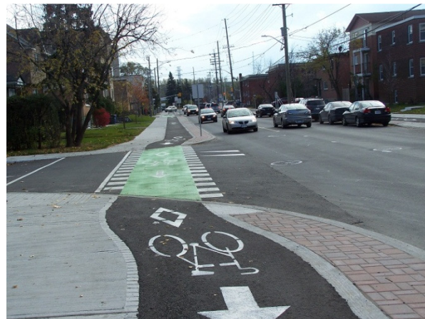
Figure 10: Pavement markings at unsignalised intersection
