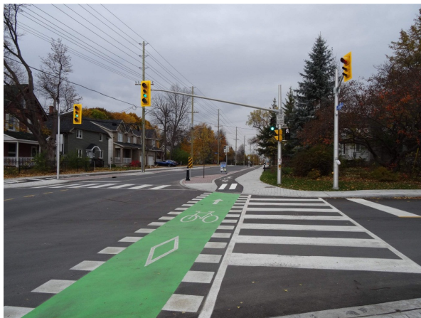
Figure 9: Pavement markings at signalised intersection
