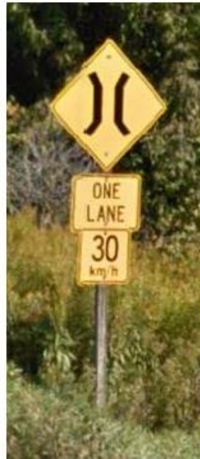
WA-7T Augmenting Narrow Structure Sign on Conc. Road 1 at CPR
