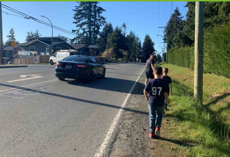
Portions of Metral Drive provided only gravel shoulders and wide vehicle lanes prior to the re-design
