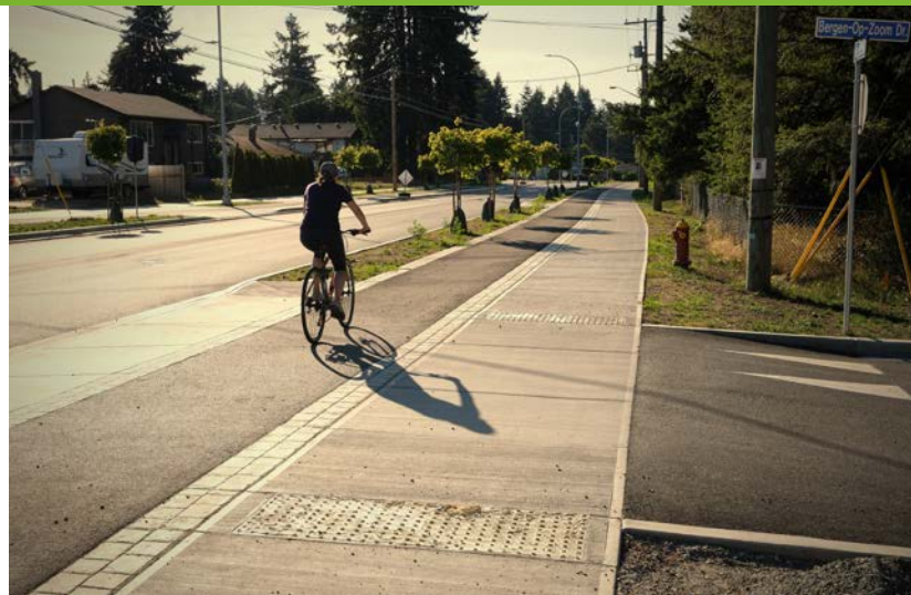
Metral Drive now showcases modal separation and continuous sidewalks and bike lanes
