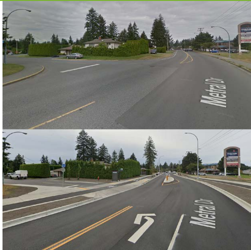
Google Street View before & after showing the new raised local intersections on Metral Drive
