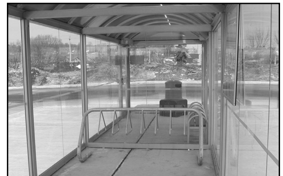
Figure 3-37. Bicycle parking may be integrated into waiting areas providing weather-protected parking. Source: JoAnn Woodhall, Region of Waterloo
