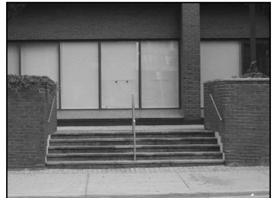
Figure 3-24. Steps leading to building entrances are discouraged as they present problems for people who have mobility impairments.
