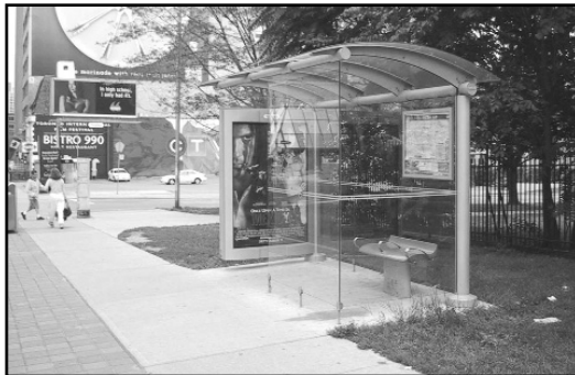
Figure 3-38. Bus shelter is located away from street protecting passengers from splashing and maintaining clearance for pedestrians on sidewalk.
