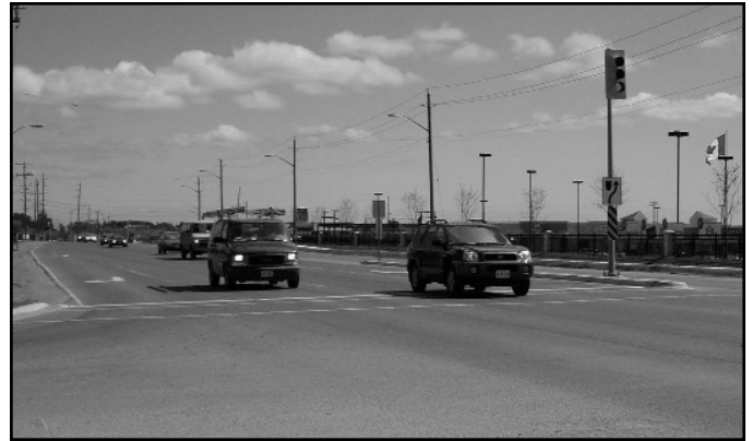
Figure 3-47. The structure and density of land-uses has a major impact on the attractiveness and convenience of more sustainable transportation modes.
