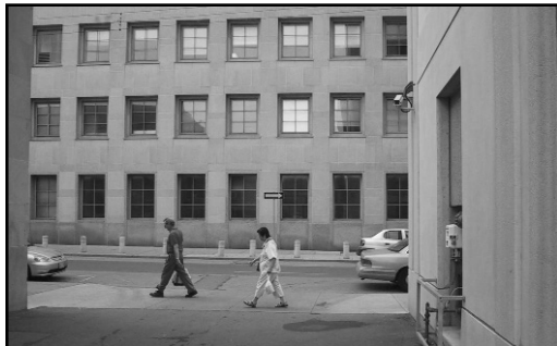
Figure 2-3. Avoid designs where vehicle drivers exiting from driveways cannot see approaching pedestrians, as illustrated.
