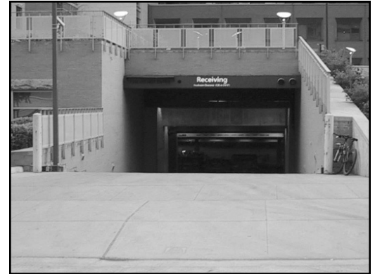
Figure 3-22. On larger sites in urban settings, loading areas can be located underground to minimize impacts on pedestrians and cyclists. Pedestrians and cyclists should be clearly visible from the loading ramp exit. Source: IBI Group
