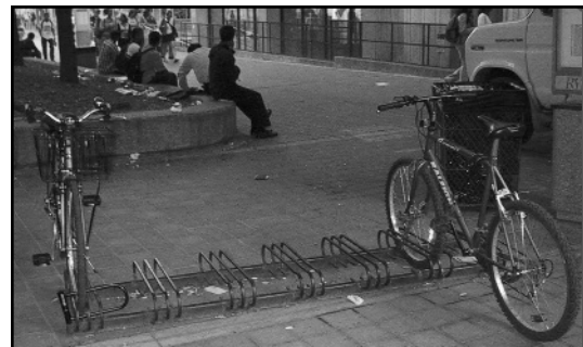
Figure 3-43. Unacceptable bike rack design (frame of bike cannot be secured). Source: IBI Group
